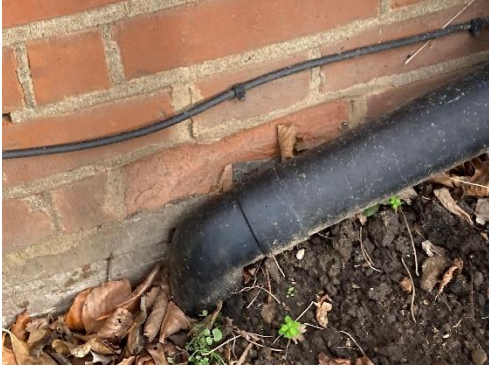
10 Spalled masonry
