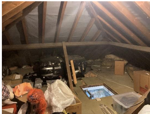
20 Main roof structure
