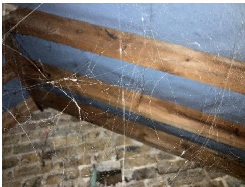
21 Rear addition roof structure
