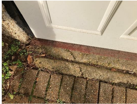
34 Cracked threshold
